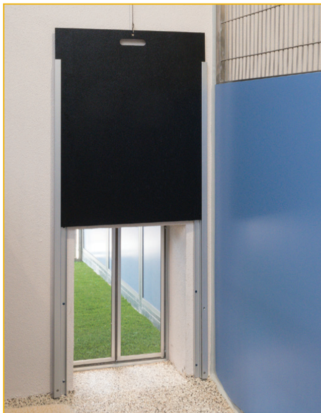
Cover panel raised to open position by cable system.
